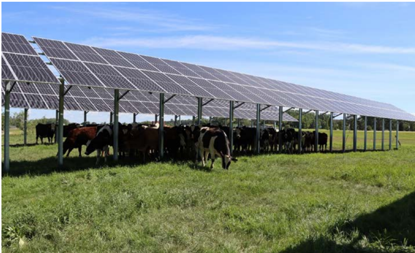
Fig. 1: The 500-kW solar photovoltaic ground-mounted system for solar shading at the University of Minnesota West Central Research and Outreach Center in Morris, Minnesota, USA.
